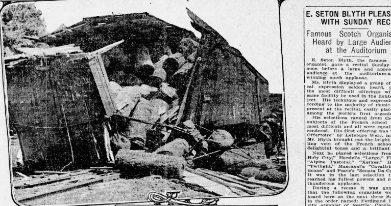
Upper picture shows rear Pullman as it was telescoped by freight engine. Through the window can be seen point where Mrs. R. T. Cresce was caught in wreckage. It required an hour's work to extricate her. Mrs. George Matheson, of Atlanta, was also in the rear of the last Pullman and received serious injuries. In the lower picture one of the smashed freight cars and its scattered contents are shown.
